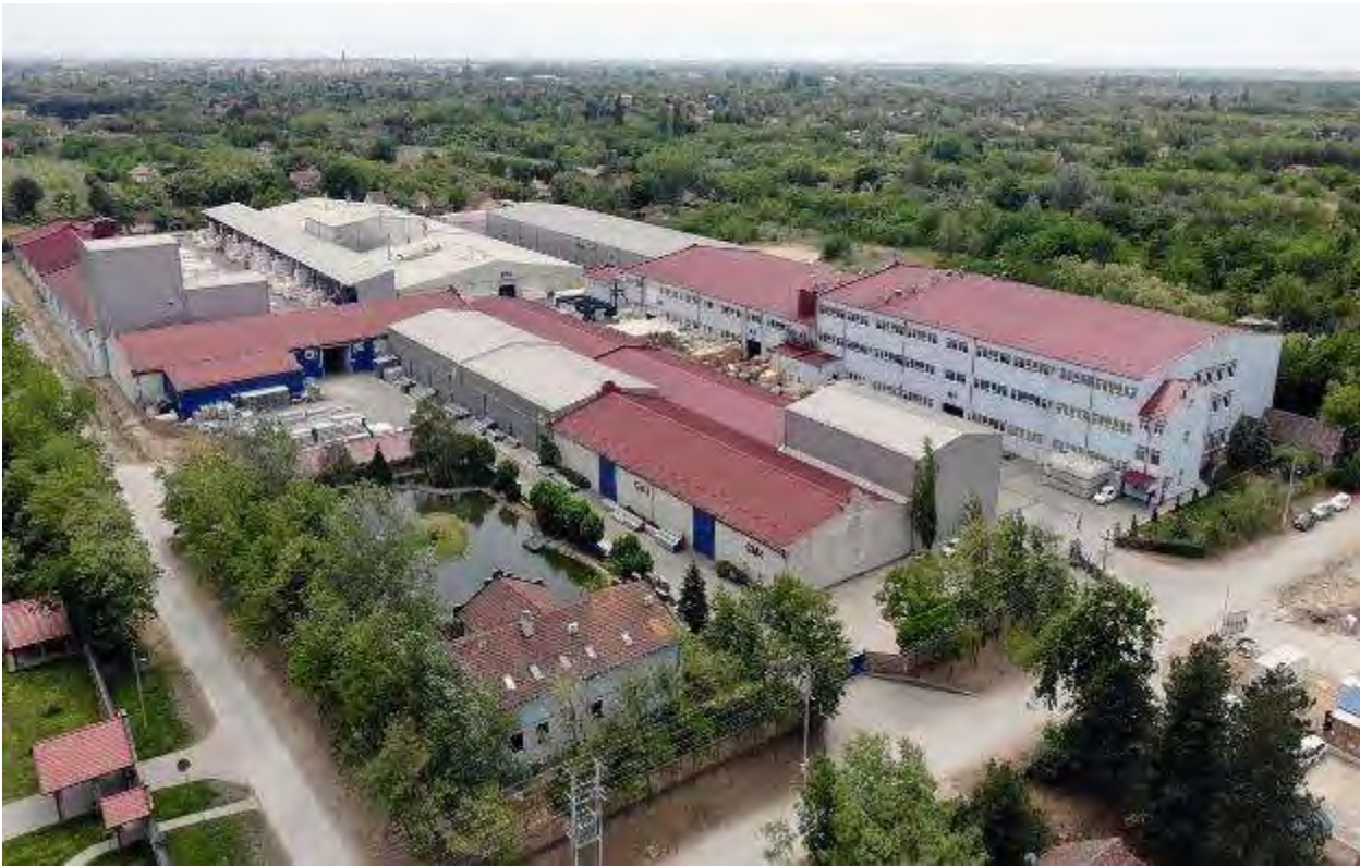
Subotica – EPS plant
