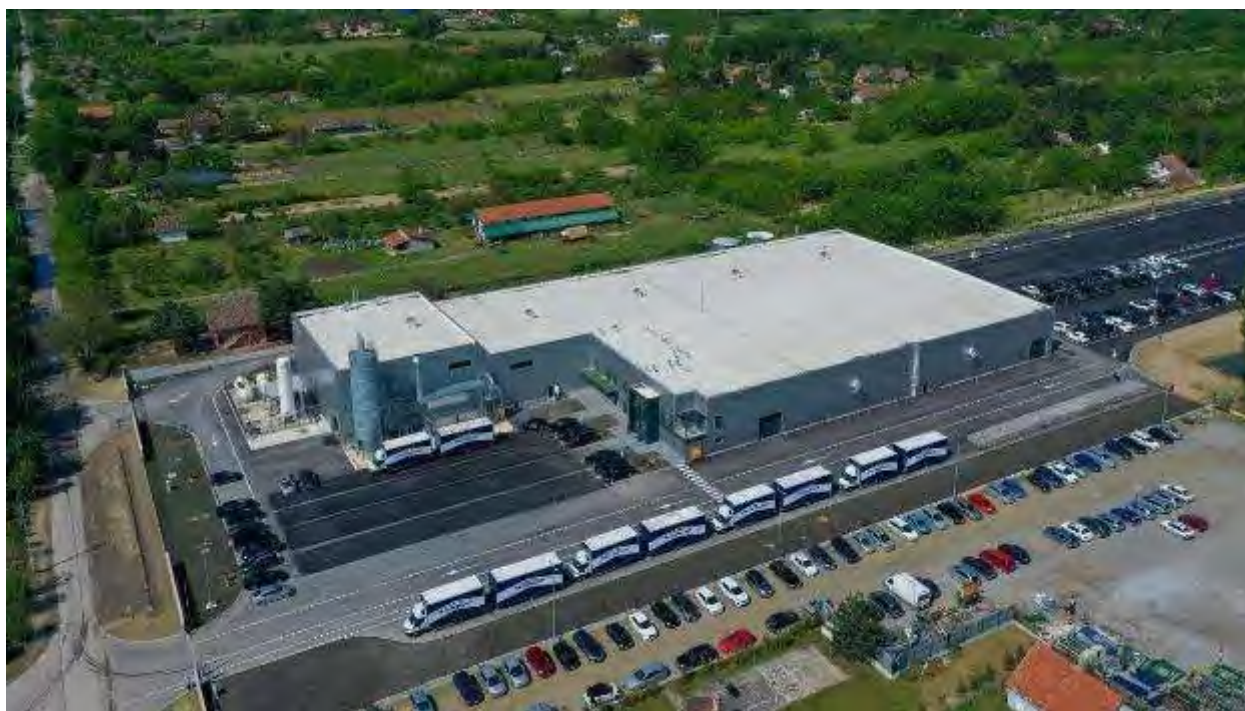
Subotica – XPS plant
